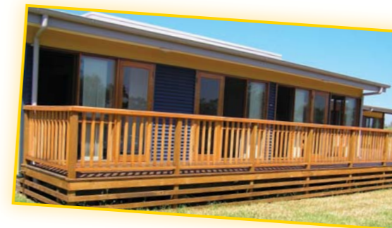
The new La Perouse Community Health Centre
